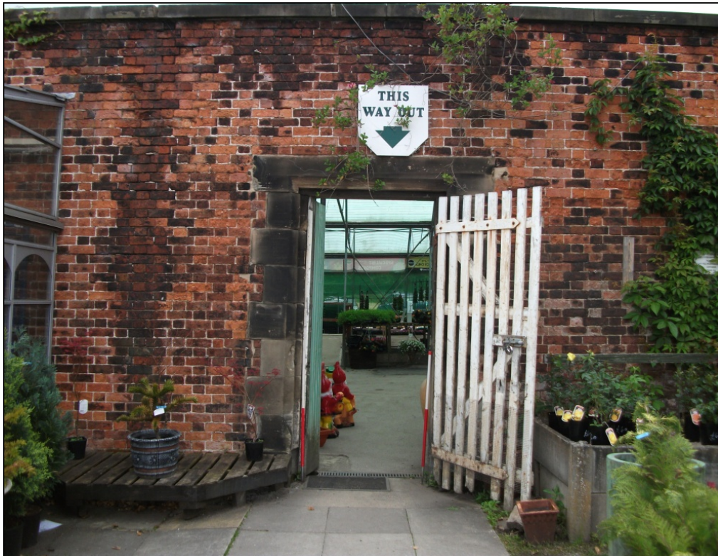
Fig 29: View of doorway at the northern end of the Western Elevation, looking W.
