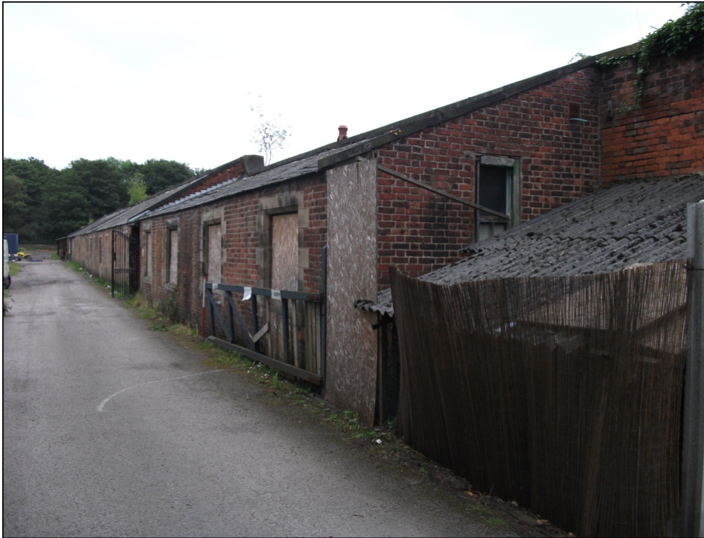
Fig 9: View of Boiler House and Potting Sheds along the North Elevation of the garden, looking SE
