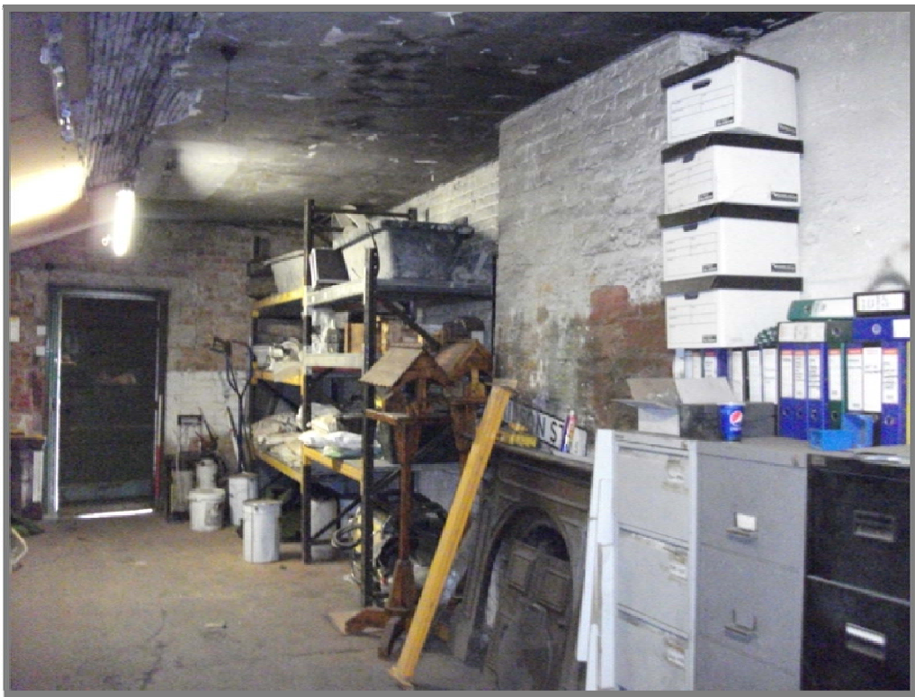
Fig 41: Interior view of the Boiler House along the gardens Northern Elevation, looking E.
