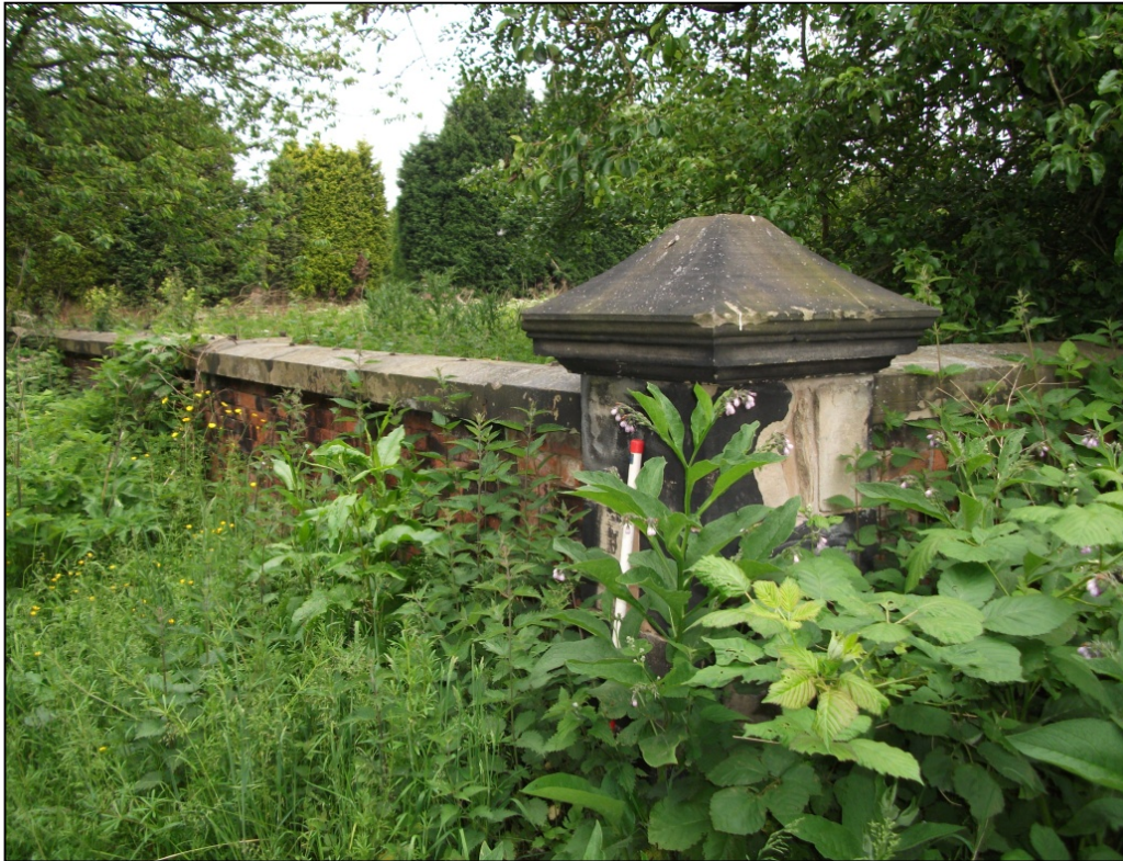
Fig 23: Stone pilaster at the south-east corner of the garden, looking NW
