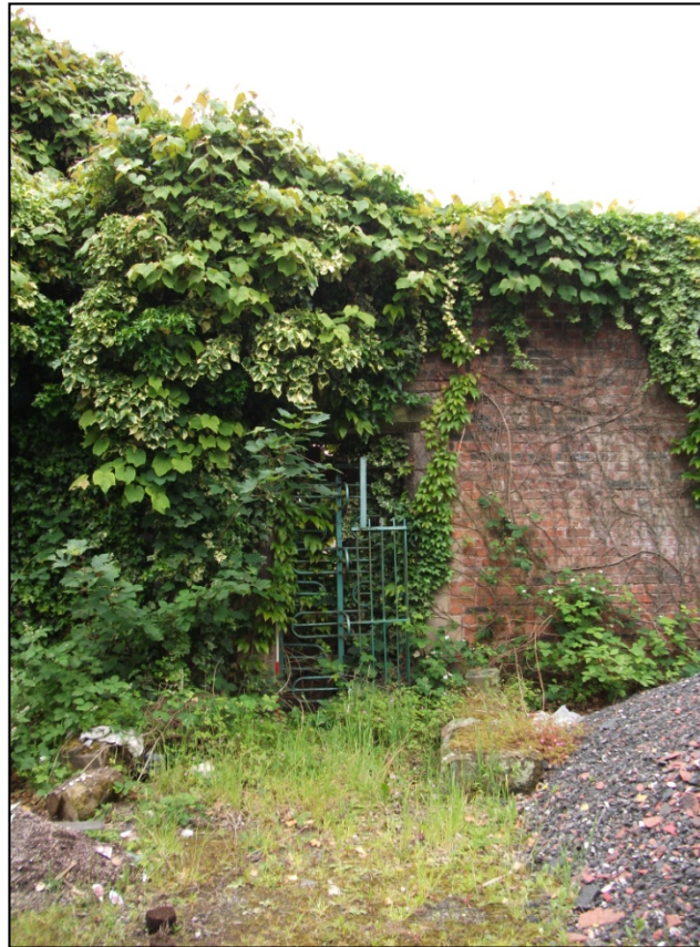
Fig 17: Doorway with a turnstile at the northern end of the gardens Eastern Elevation, looking W.
