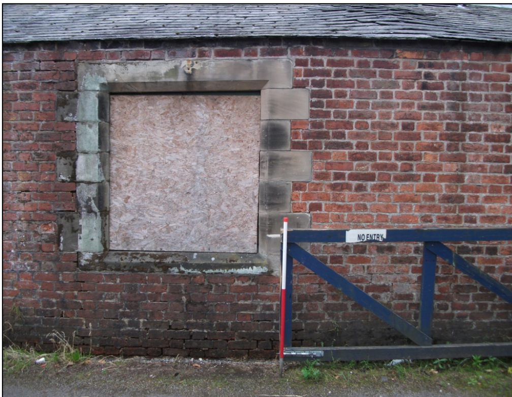
Fig 10: Window on North Elevation of the Boiler House, looking S.
