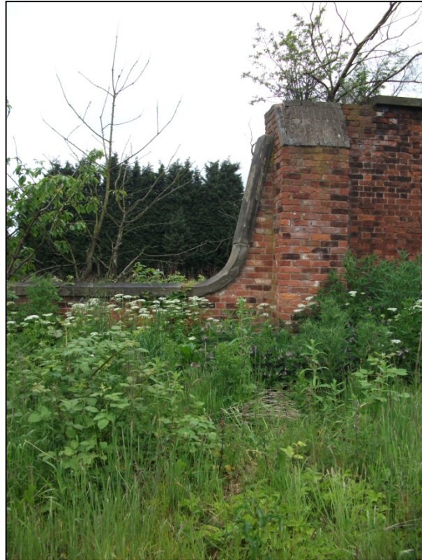
Fig 21: Central doorway along North Elevation of the Potting Sheds, looking S.
