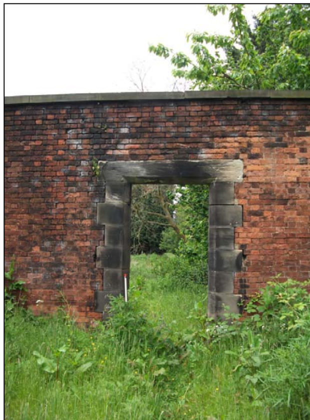
Fig 20: Central doorway along gardens Eastern Elevation, looking W.
