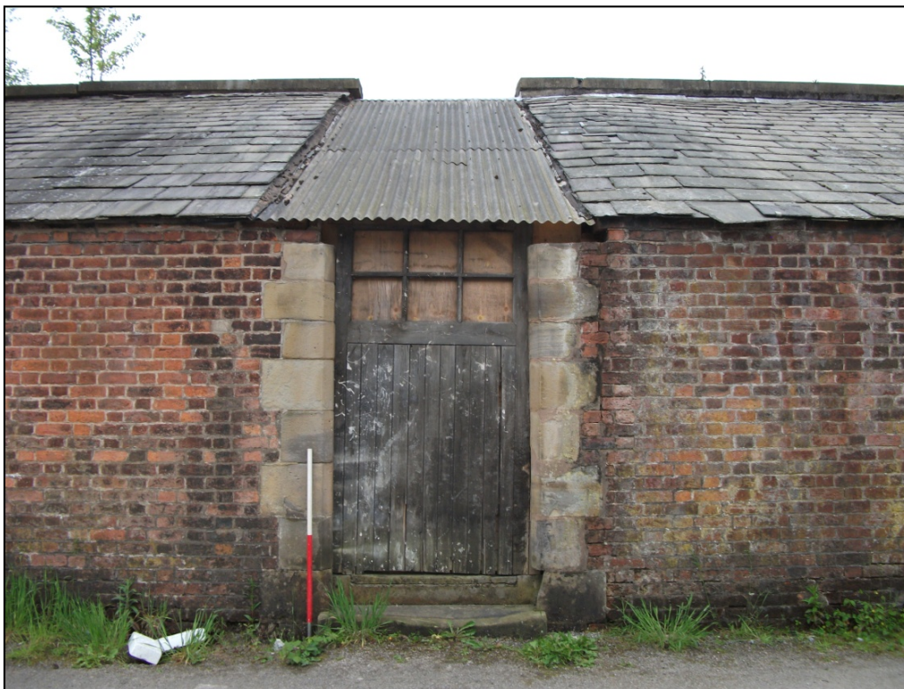
Fig 12: Central doorway along North Elevation of the Potting Sheds, looking S.
