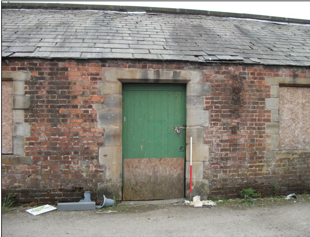
Fig 11: Western doorway along Northern Elevation of the Potting Sheds, looking SW.
