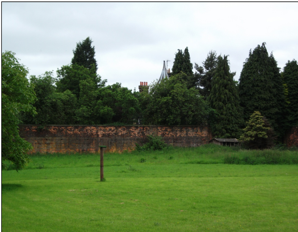
Fig 35: View of the inner face of the gardens Western Elevation, looking W.
