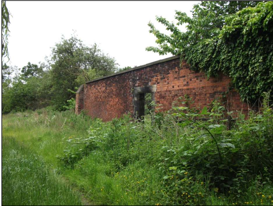
Fig 19: Southern half of gardens Eastern Elevation, looking SW.
