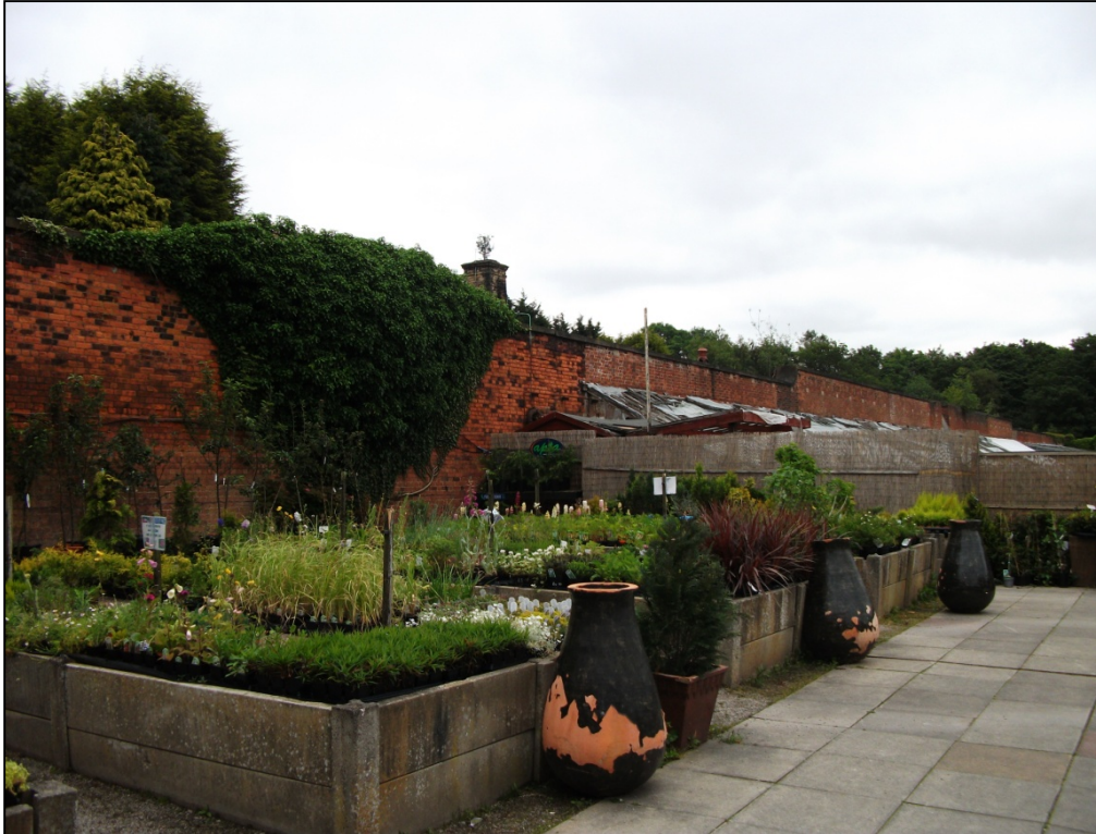
Fig 32: View of inner face of the gardens Northern Elevation, looking NE.
