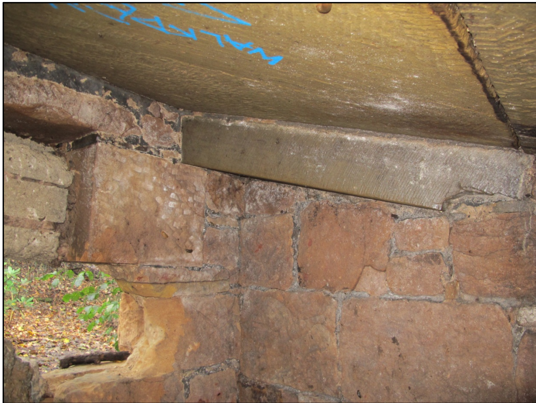
Fig. 19 – Shot of stone lined approach chamber and partially blocked entrance. Looking North-east.
