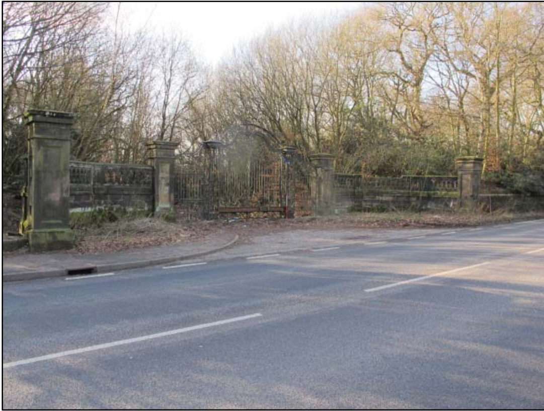
Fig. 8 – Wide shot of gates. Looking South-west.
