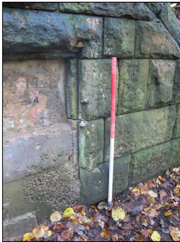
Fig. 21 – Detail of blocked doorway in northern elevation of ice house. Looking south.
