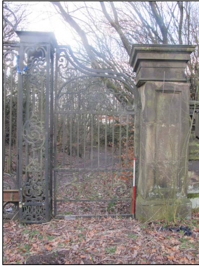
Fig. 10 – Shot of western pedestrian gate and stone pillar. Looking south.
