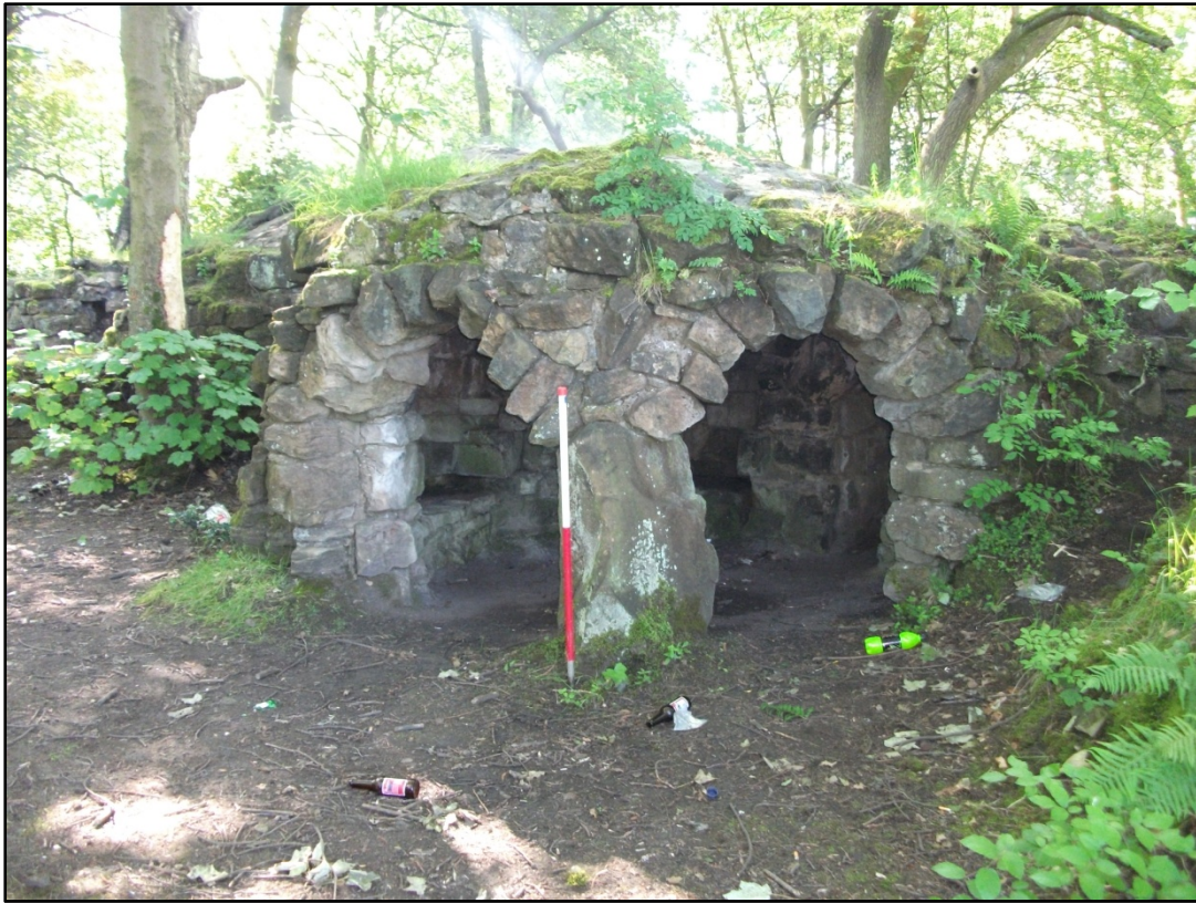
Fig. 14 – Shot of western small chamber entrance. Looking east.
