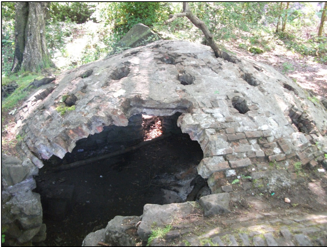
Fig. 15 – Shot of Grotto's brick roof. Looking south-east.
