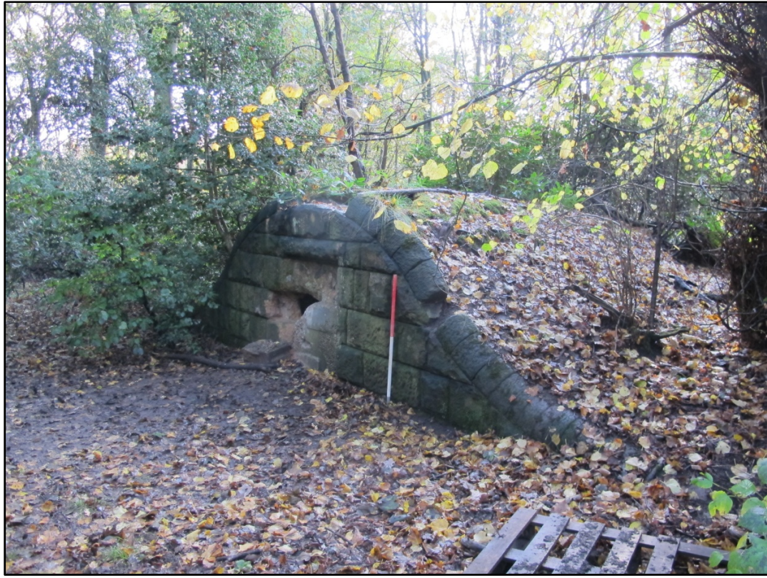
Fig. 20 – Shot of northern elevation of ice house. Looking south-east.
