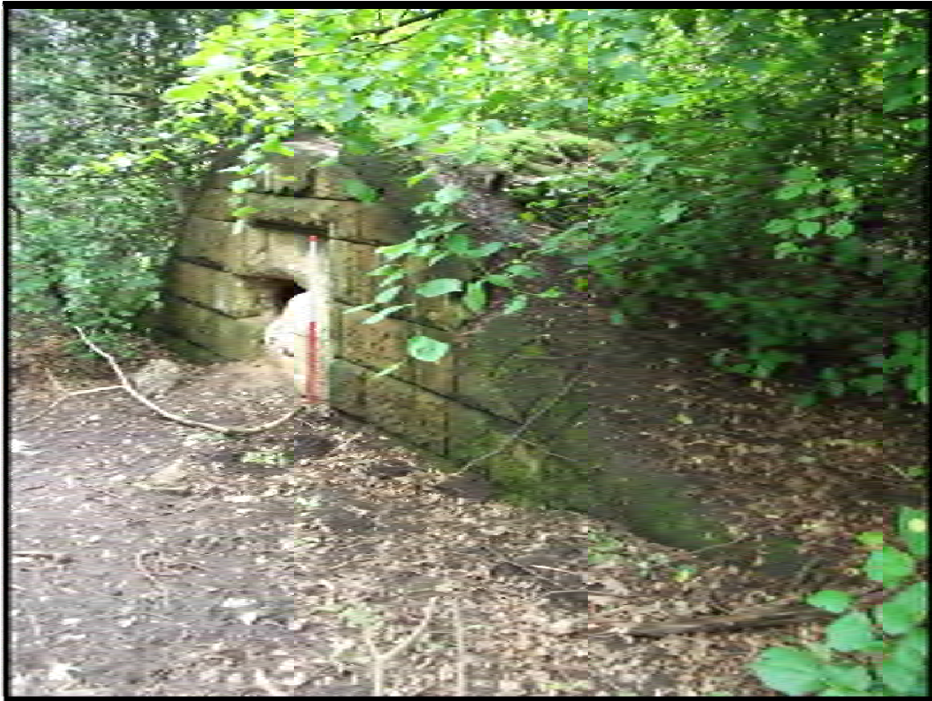
Fig 23: View of the New Hall Ice House (Site 26), looking South-East.
