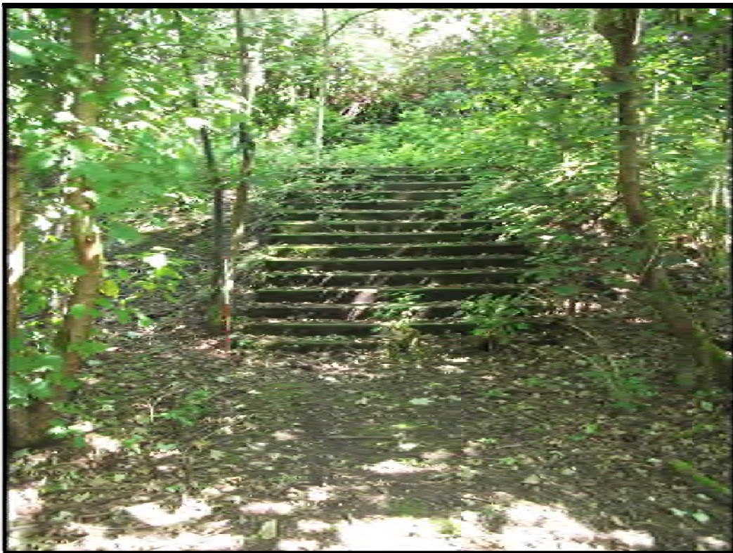
Fig 24: View of Steps (Site 30) leading to the Leigh Road Footbridge (Site 29), looking North.
