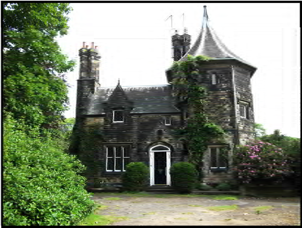
Fig 15: View of the Garden Cottage south elevation ( Site 1 ), looking North.
