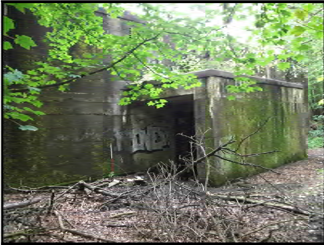
Fig 25: View of Concrete Bunkers southern elevation ( Site 32 ), looking North-East.
