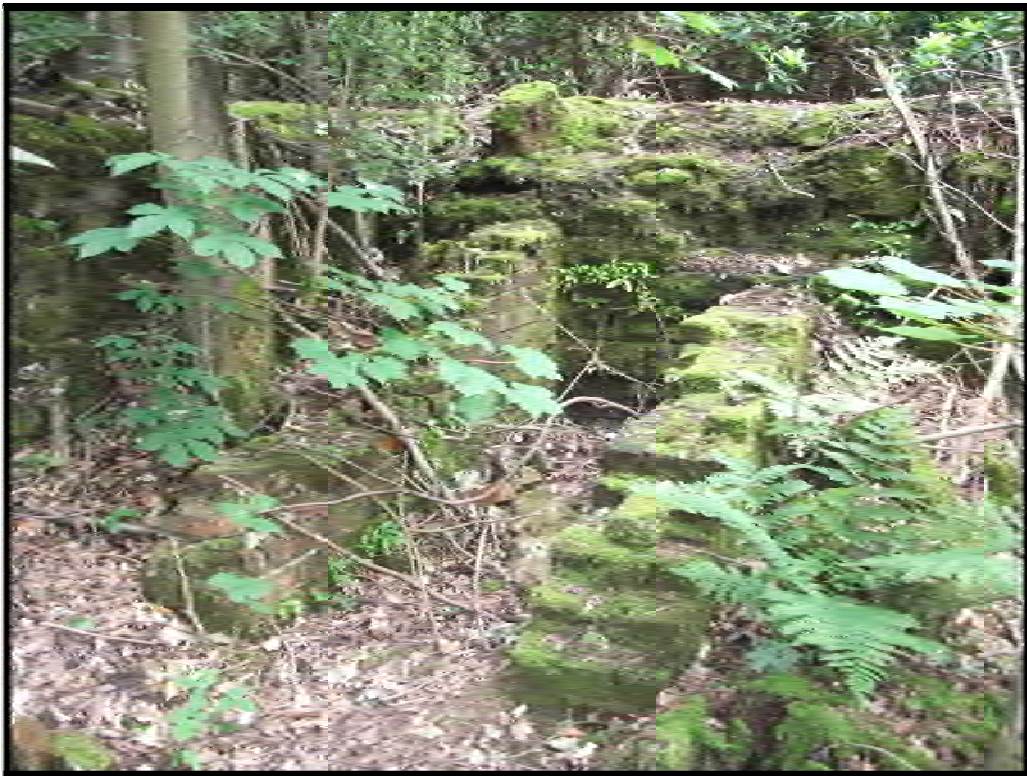
Fig 30: Remains of Steps leading down from the New Hall Gardens Main Terrace (Site 33b), looking North-East.
