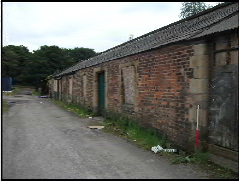
Fig 17: View of Potting Sheds (Site 6), looking East.
