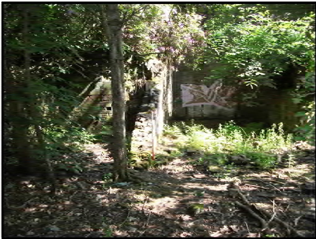
Fig 22: Remains of New Hall Pump House / Fire Station ( Site 27 ), looking North.
